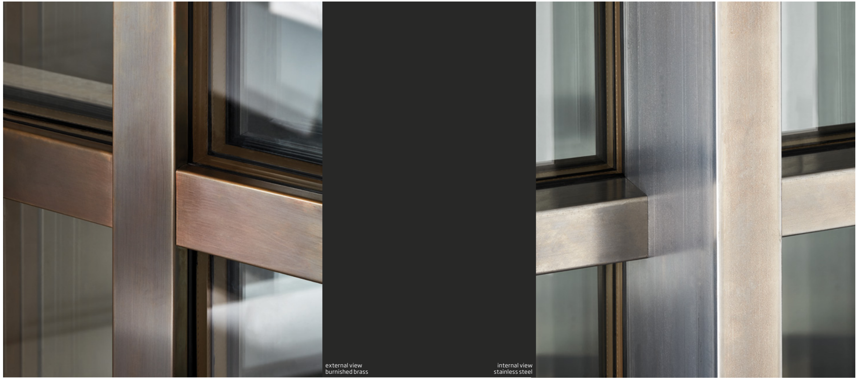
4F 1 façade section, external view, with covers in burnished brass and internal view in scotch brite stainless steel.
